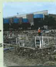
Work continues on the new Farmers Branch Aquatics Center
